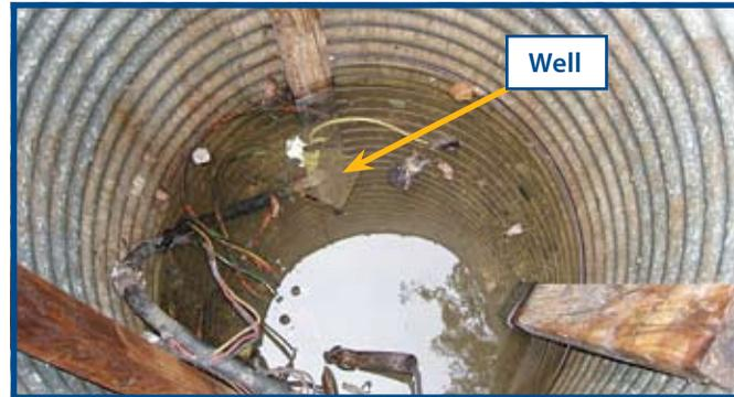
Figure 3. Water and debris in well pit
