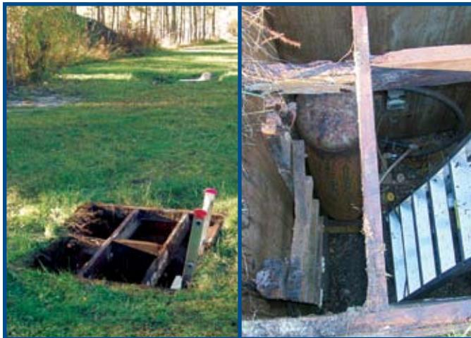
Figure 1. Well pit with wooden cribbing
