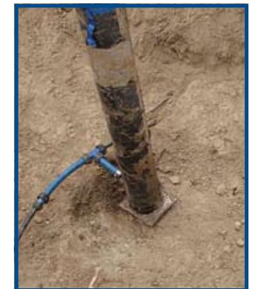
Figure 6. Pitless adapter installed below frost line
