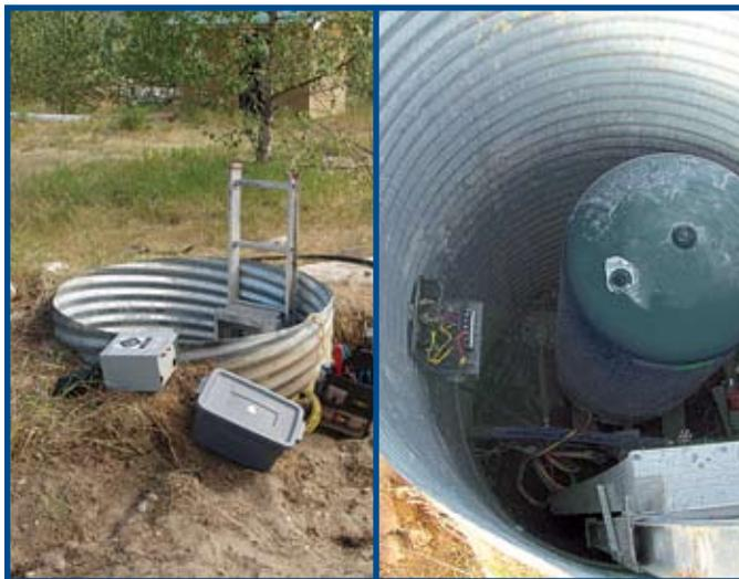
Figure 2. Well pit with metal cribbing
