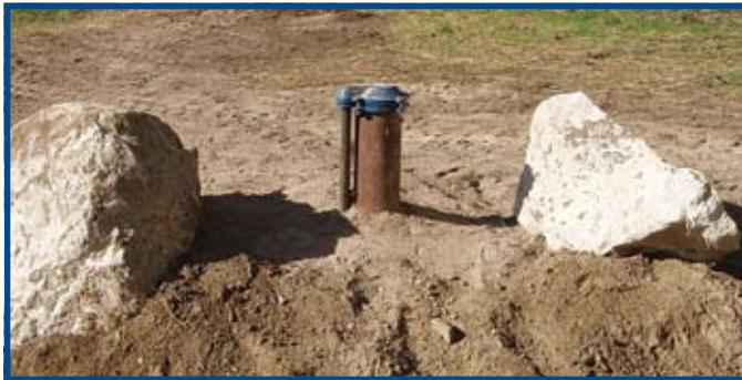
Figure 8. Grading around well head to protect well
