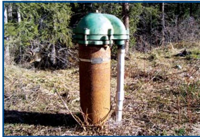
Figure 9. Secure well cap
